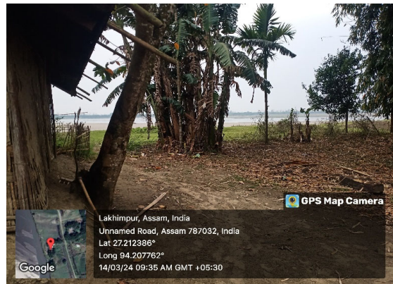
(d) Riverbank proximity of a household structure in Lakhimpur. The precarious location reflects the compulsion of landless households to settle on flood-exposed land, underlining the intersection of natural capital loss and structural landlessness.
