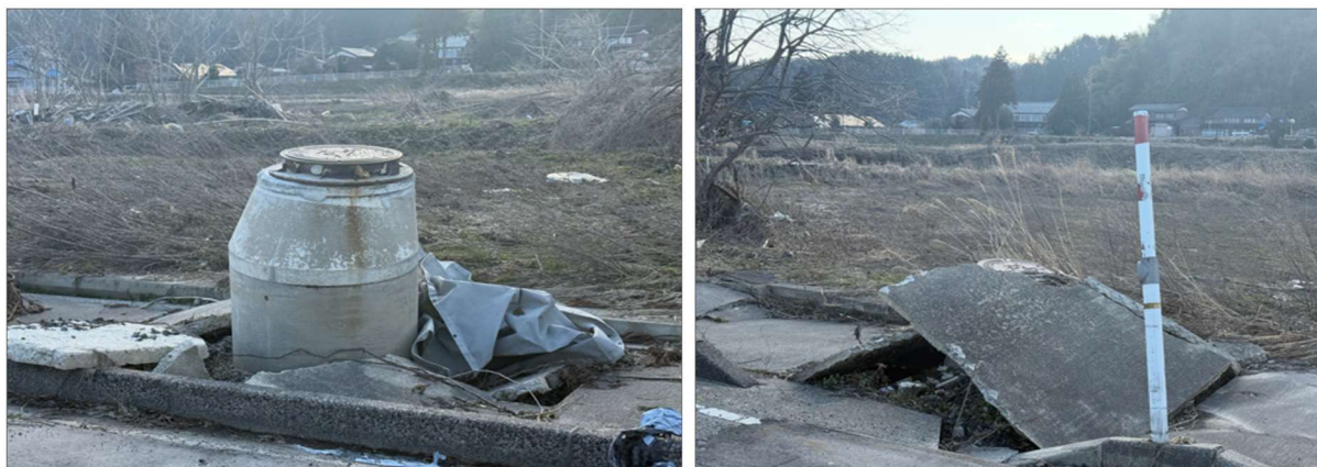
Figure 4. Damage to underground water infrastructure in Suzu City, after the 2024 Noto Peninsula Earthquake (March 2025).
