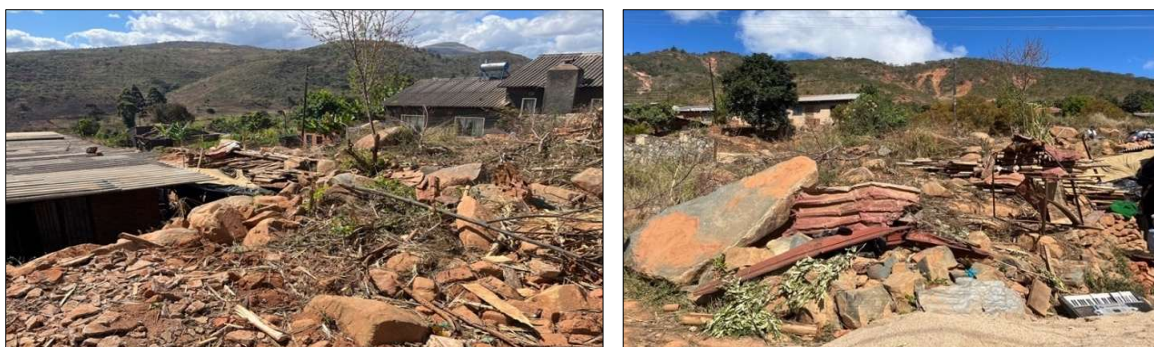
Figure 2. Ongoing landslide damage in Chimanimani Ward 15 (Author, 2023)
