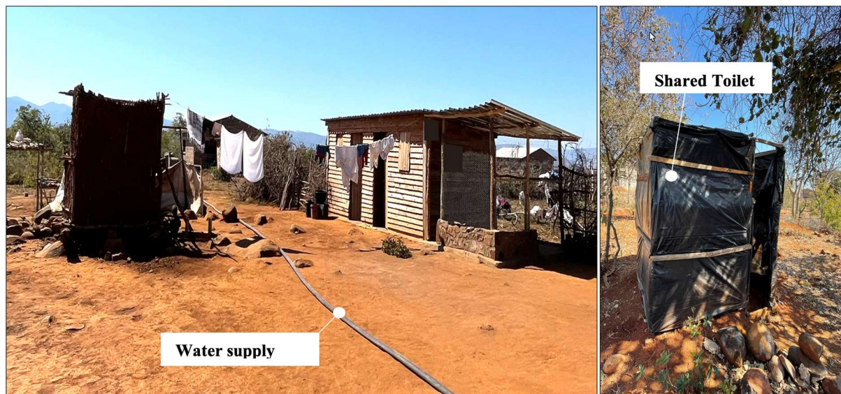
Figure 11. Phase 2 permeant housing - West End Ward 7 (Photography by Author, 2023)
