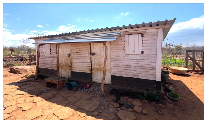
Figure 8. Modified Phase 1 unit - West End -Ward 7 (Photography by Author, 2023)
