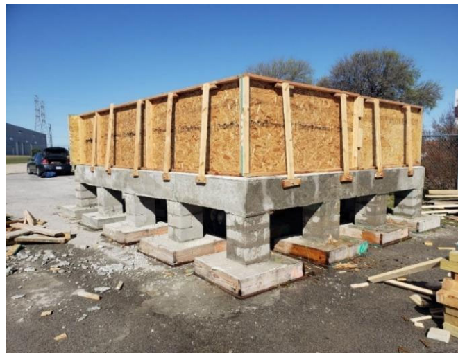
Figure 5. Experimental elevated slab specimen
